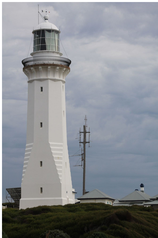
Green Cape Lighthouse Photo by RW
