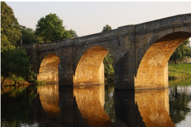
A bridge over the North Tyne
