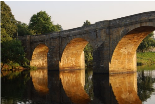
A bridge over the North Tyne
